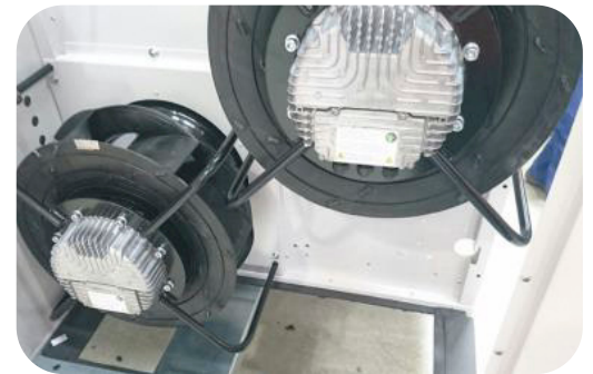
EC motor fans in VECTIOS rooftop units
